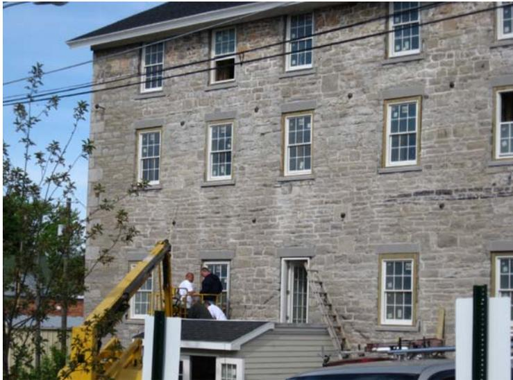
Replacement windows are installed in a historic structure. Modern window design and materials incorporate the historic sash pattern (6 over 6 double hung sash).
